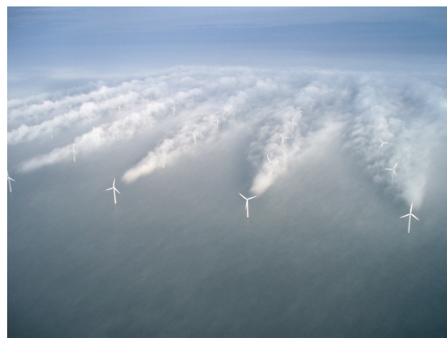
Figure 1: Horns Rev wind farm in fog conditions, making visible the wake effect. Photo: Vattenfall.
